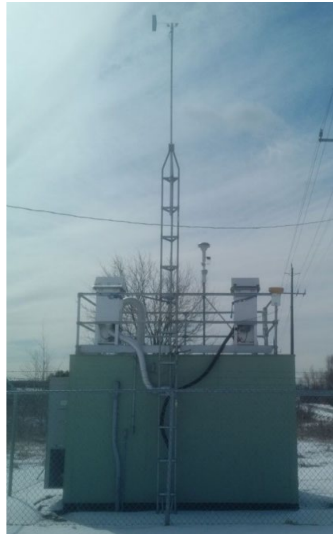
Figure 3: Rundle Road Station
